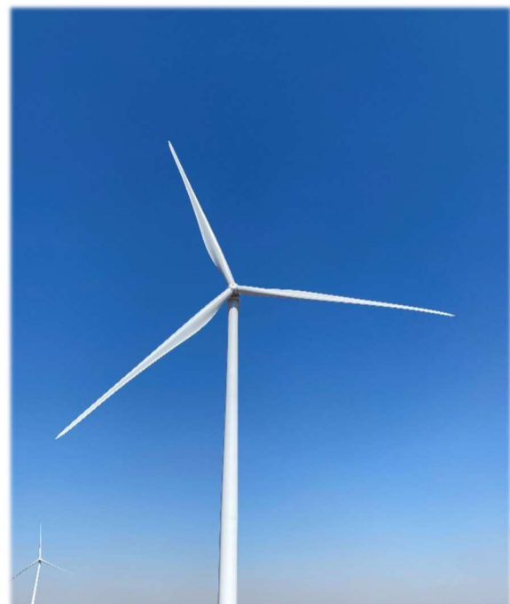
One of the 72 wind turbines at the Sundance wind farm, which began commercial operation in April 2021.
