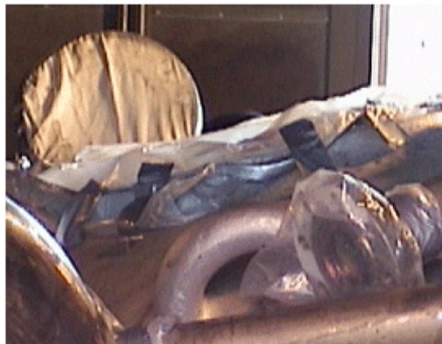
Figure 3a. Examples of FME Covers utilizing Paper, Linen and Plastic Bags (Not a Recommended Practice)
