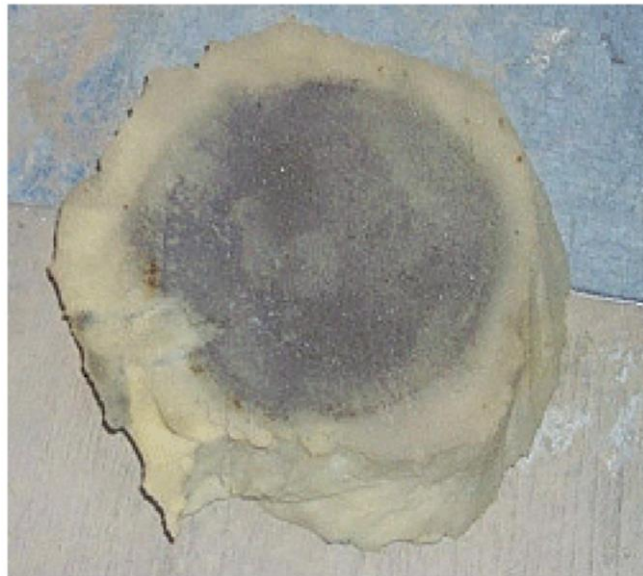
Figure 2. 12” Piece of Foam Material used as an FME Cover, Removed from a Pipe Using Air Blows (Material was not detected during visual inspections)
